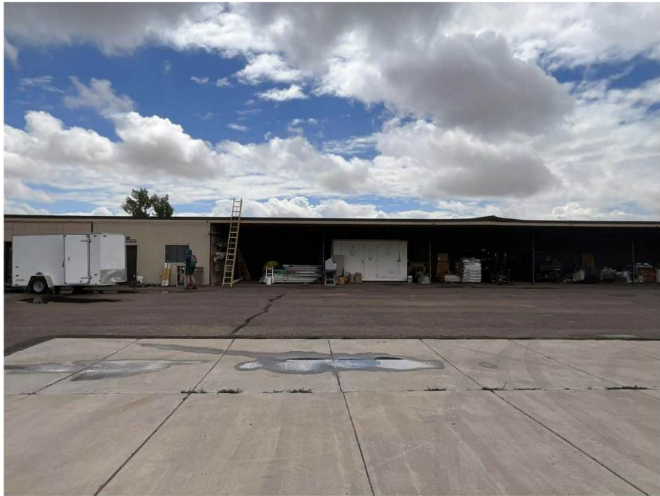
NORTH ELEVATION OF VEHICLE STORAGE BUILDING
