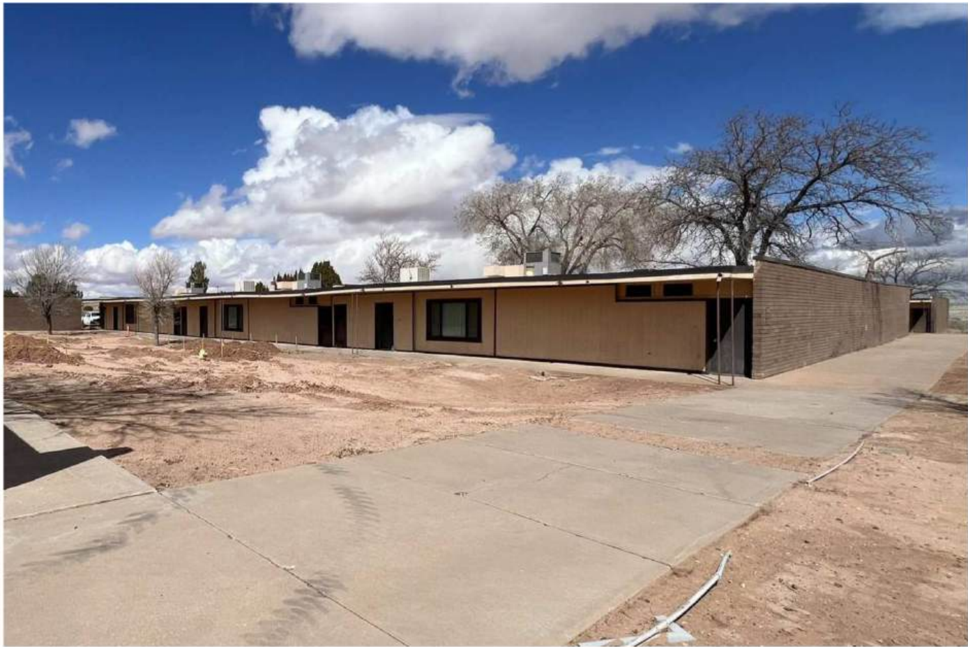
LOOKING TOWARD SOUTHWEST CORNER OF HOUSING BLOCK C
